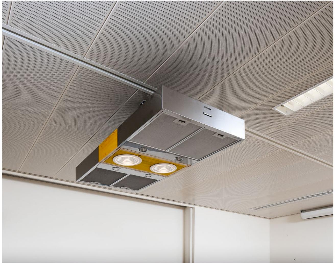
The air recirculation element consists of two standard cubic air recirculators connected together by a central box. The height of the box can be coordinated with the recirculators. Depending
