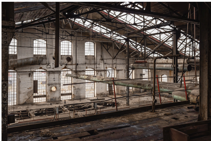
South facade of the Main Production Building / Zuckerfabrik.
