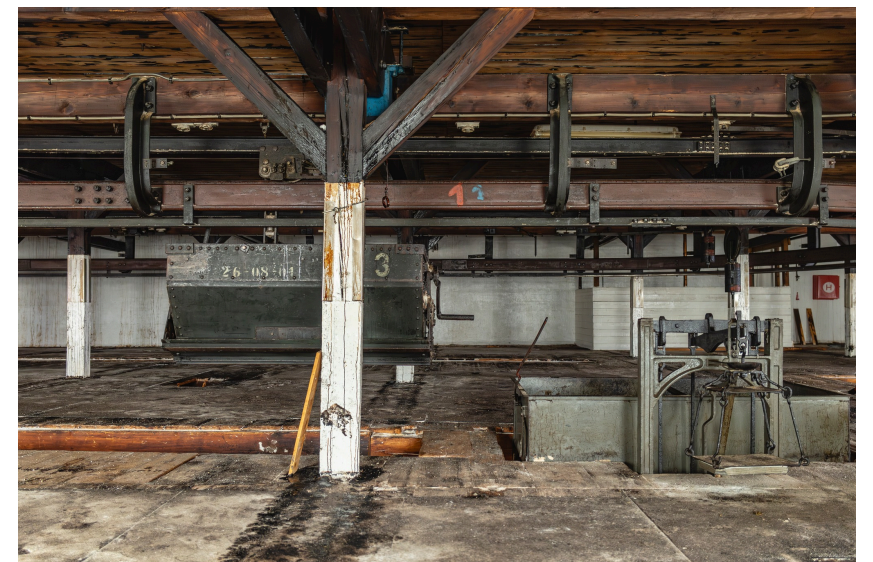
Sugar Warehouse with trolleys and a sugar weighing system.
